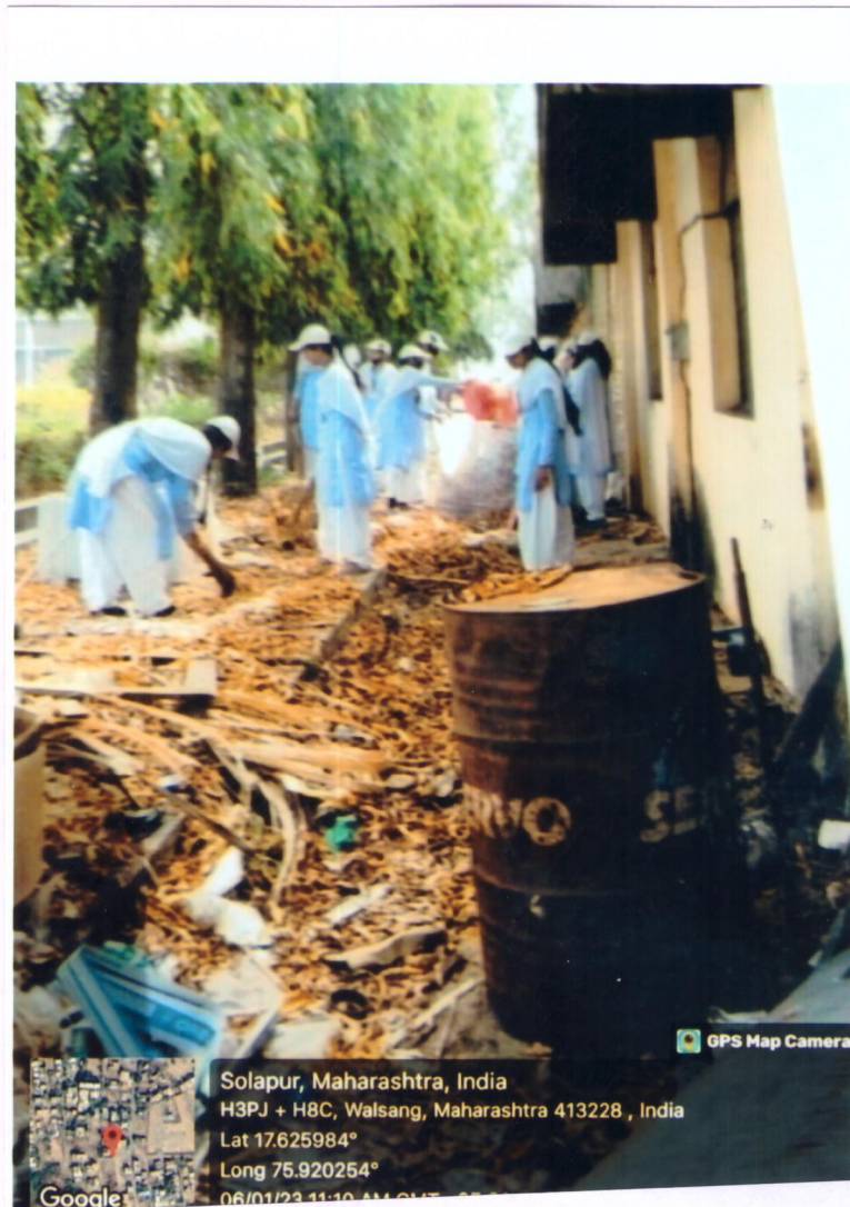
Volunteers cleaning the premises of Swami Samarth Sahakary Suthghirni
